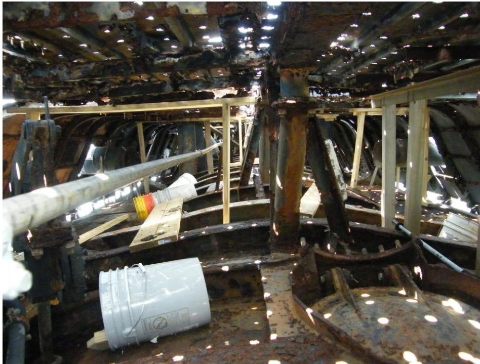
Midship area of superstructure deck being crudely supported by 2 x 4 wood planks.
