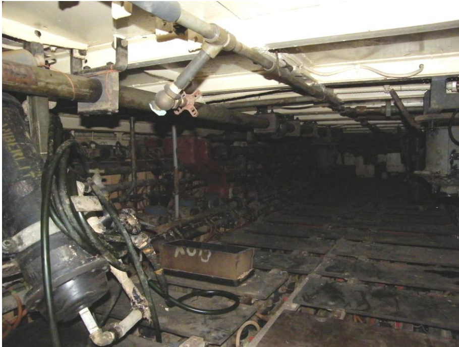
After Battery Room, looking forward to port.
