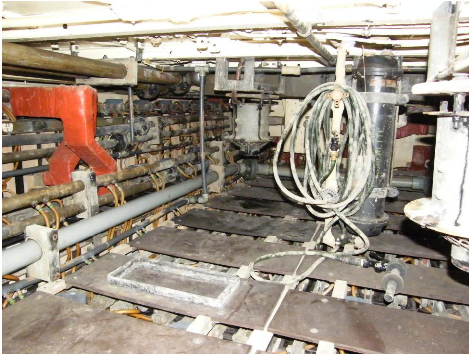
Forward Battery Room, looking forward to port. Largely original.
