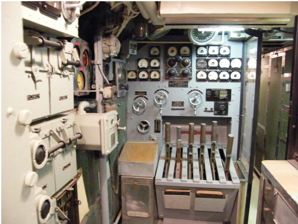
Platform Deck, Motor Control Room. Notice throttles and main panel.
