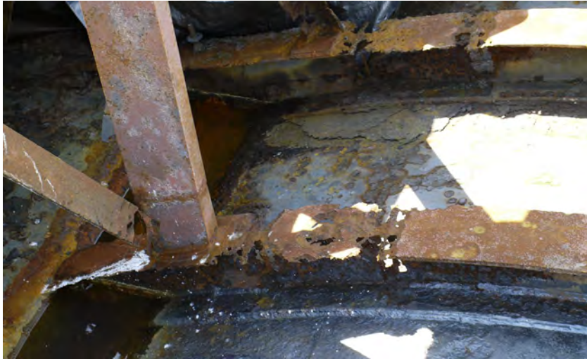
Transverse I-beams atop pressure hull.
