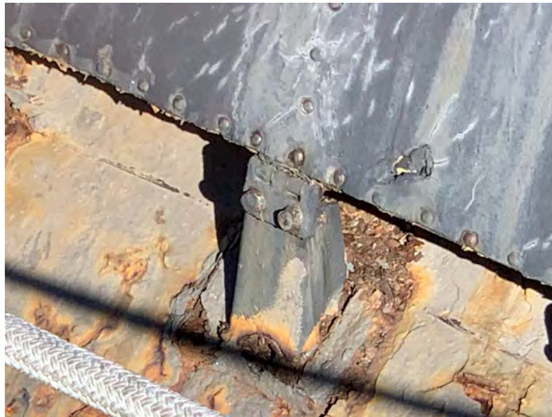
Superstructure fairing bases on hull
